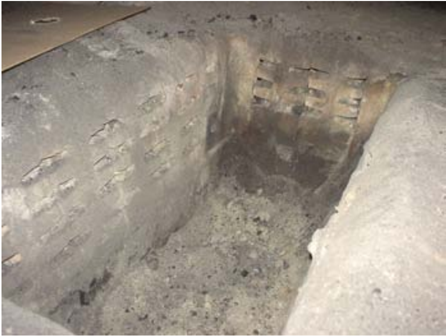
Fig.2: Standard coal grate. Air vents visible on sides. No secondary air.
