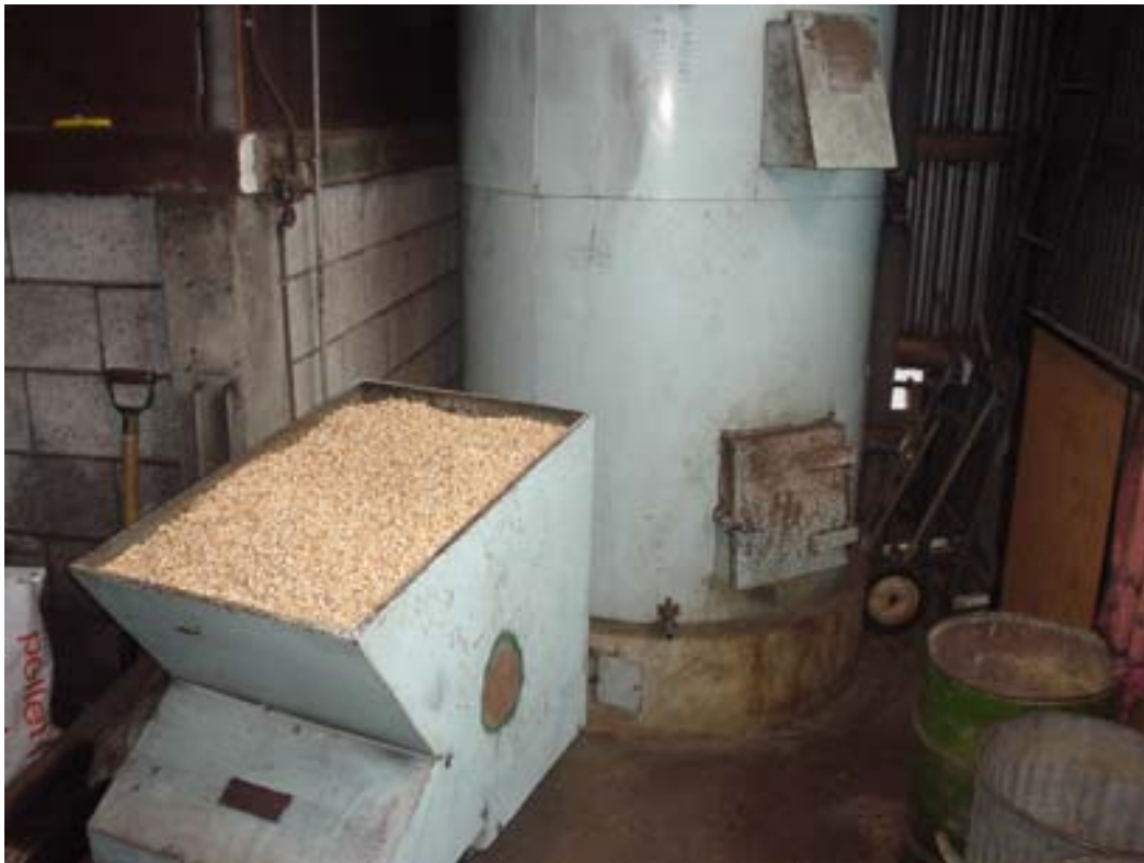
Fig.1: Test setup at Selwyn Primary School, with day hopper filled with wood pellets.
