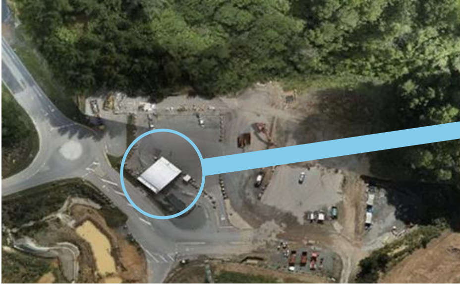
Transfer station at Silverstream landfill
