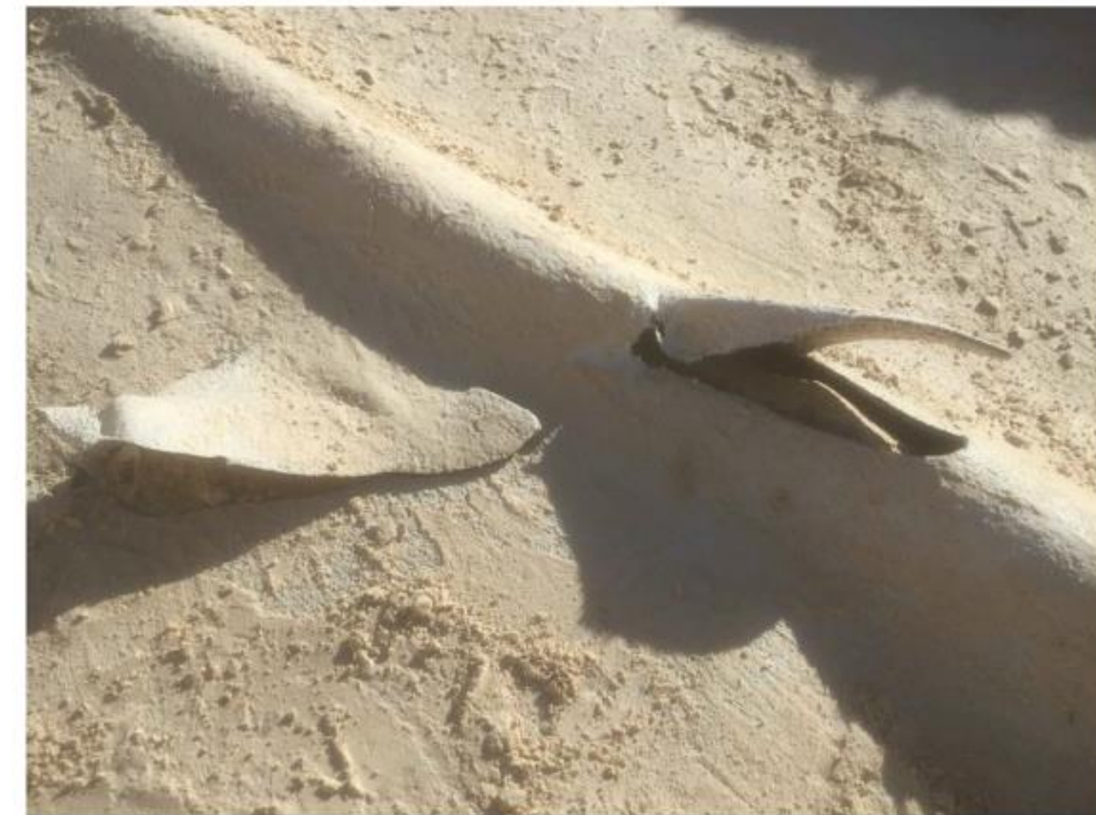
Fig. 16. Wrinkle hit by dozer blade.
