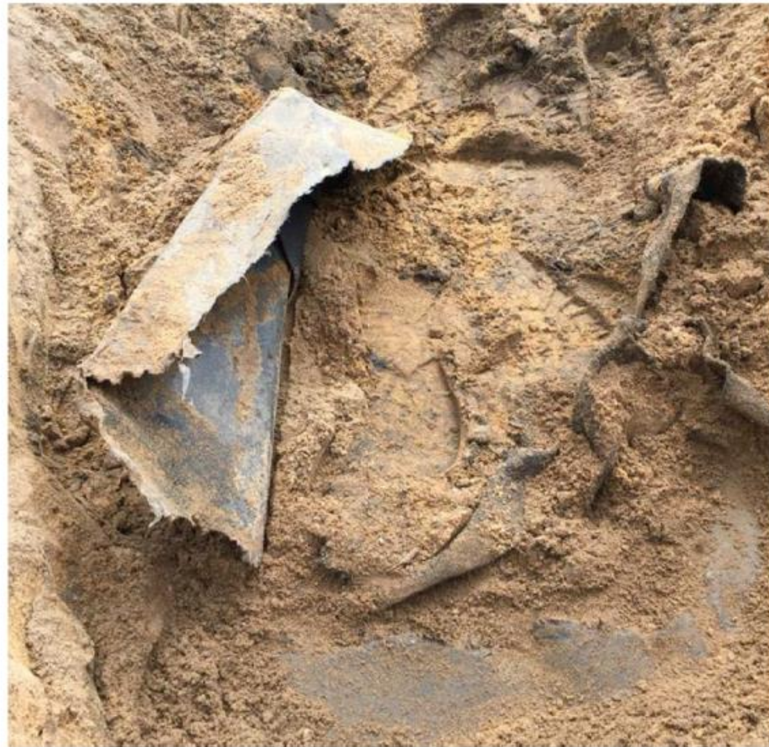
Fig. 5. Damage caused during cover material placement.
