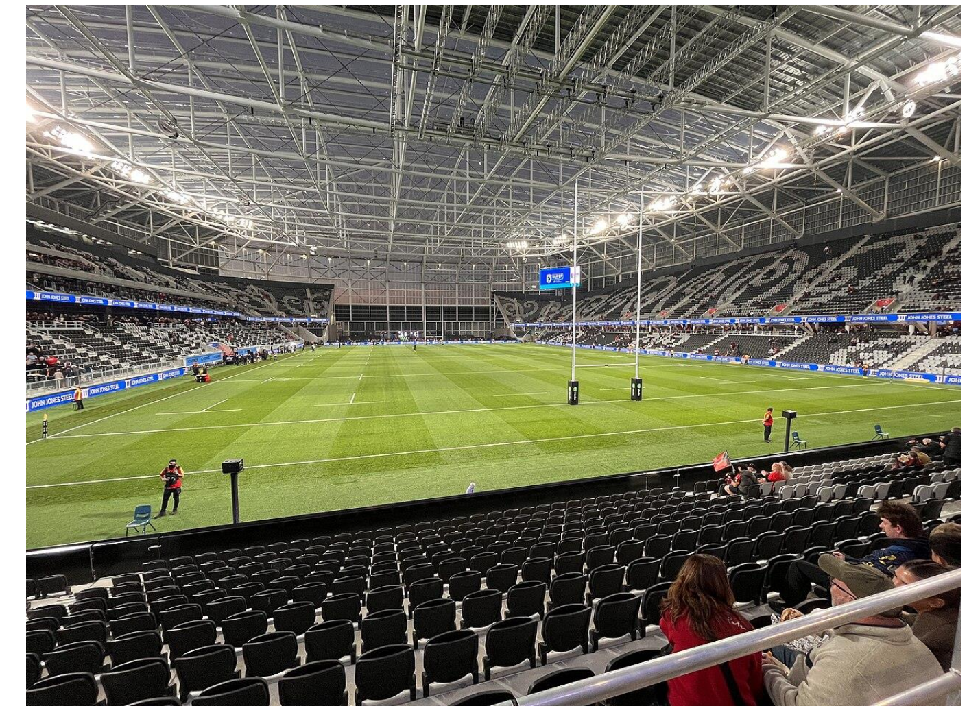
The stadium will be covered, with much of the roof made of a clear material called Ethylene Tetrafluoroethylene (ETFE), that will let natural light shine through to support turf growth: https://www.newsline.ccc.govt.nz/news/story/watch-latest-look-inside-new-stadium
