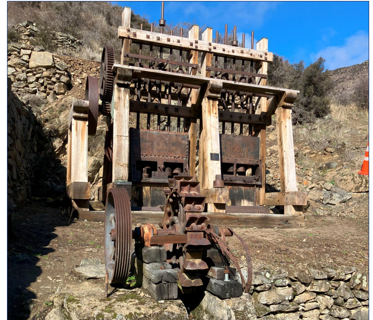
Come-In-Time historic battery and water wheel.
