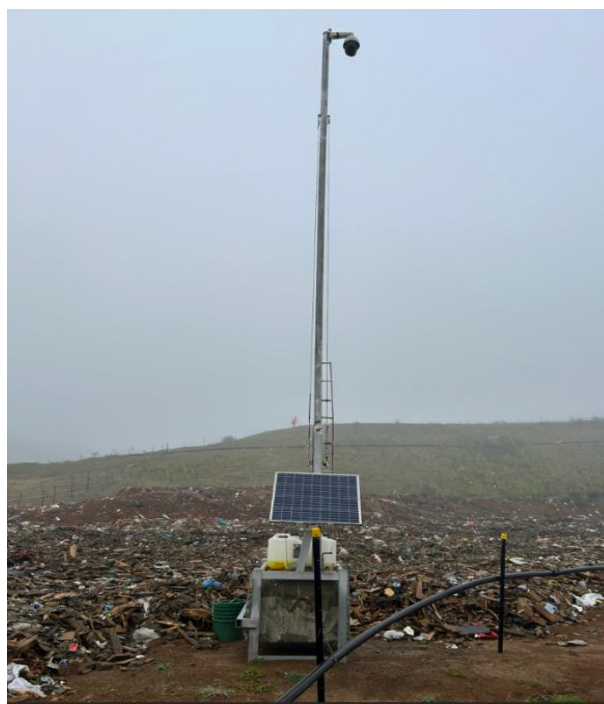
Photos: Camera system installed on 8m high poles (current installation set up).
