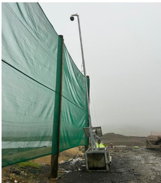
Photos: Camera system installed on 8m high poles (current installation set up).
